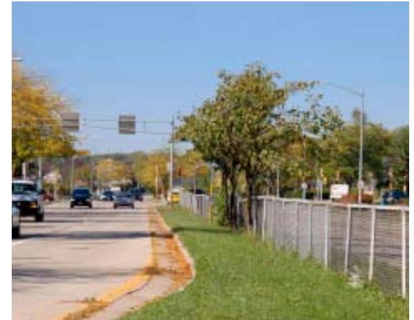
Existing chain link fence in the Northport Drive median.
